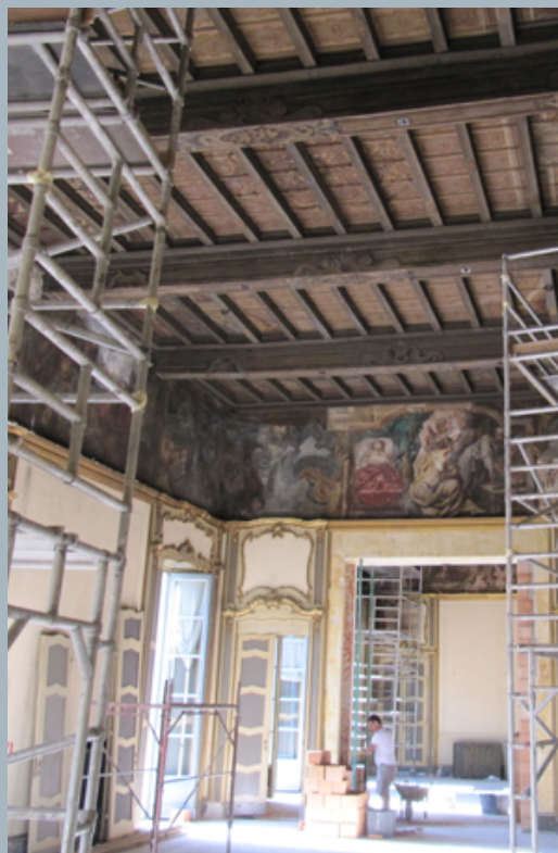
Restauro palazzo Durini (MI)
